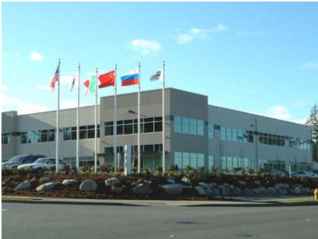
The 76,000-square-foot RSS Management/Univera Healthcare has a flexible design for multiple tenants, including the city of Lacey.
